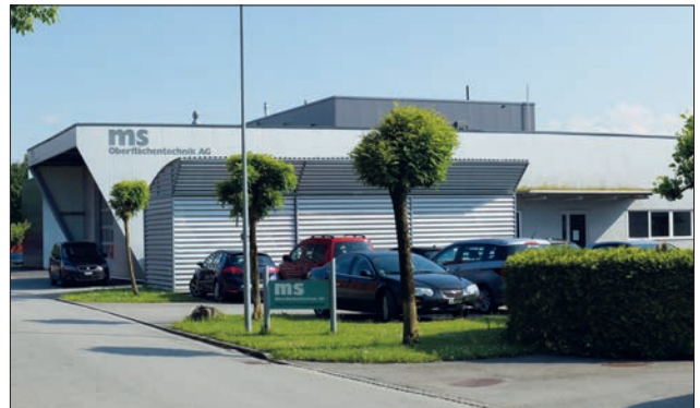
Balgach, Switzerland facility
